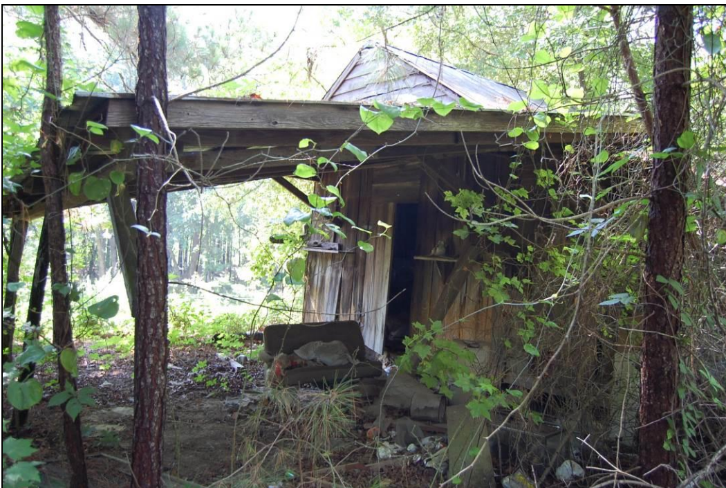
Figure 34. Shed, looking southeast
