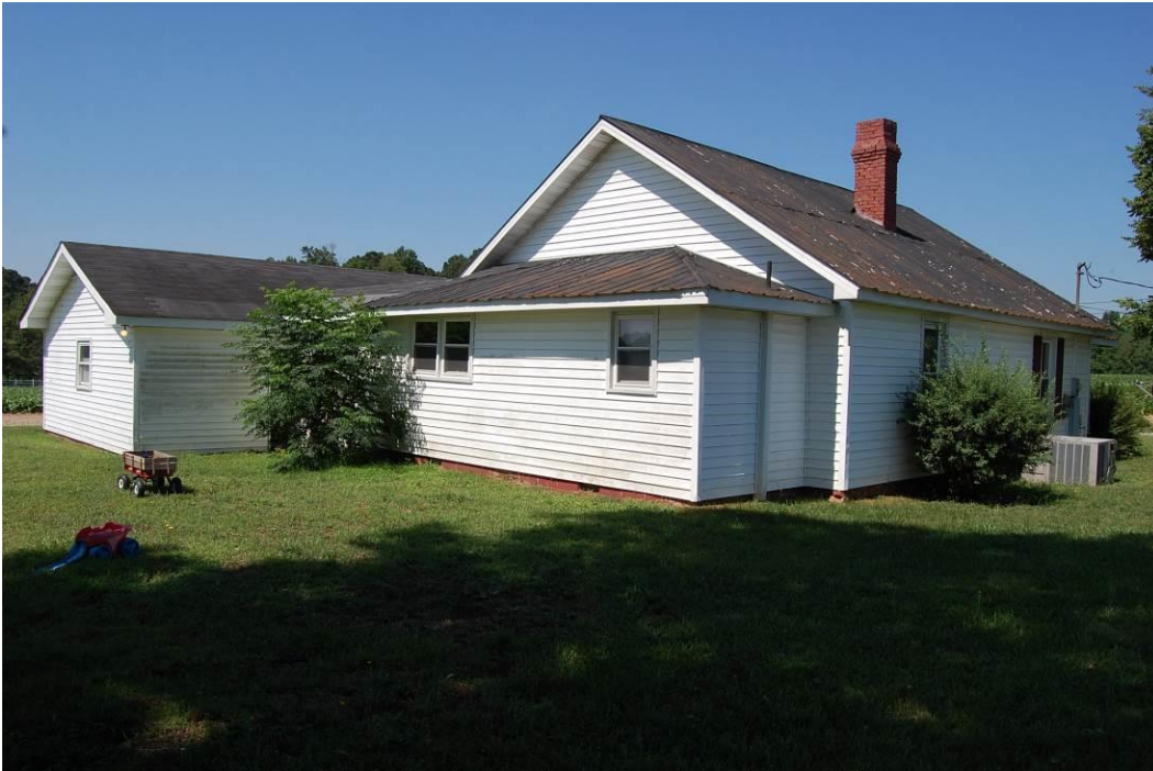
Figure 47. House, north side and east rear elevations
