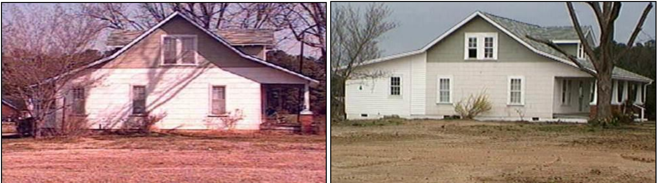
Figure 9. House, south side elevation, February 26, 1996, at left, and February 28, 1997, at right (source: Wake County tax records)
