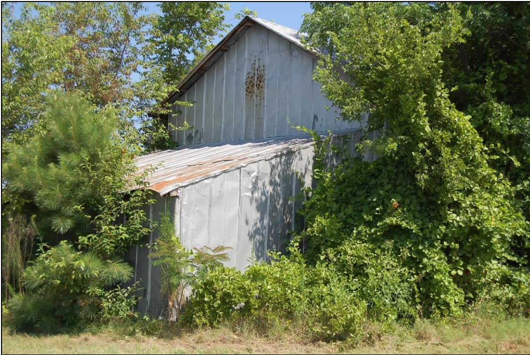
Figure 51. Looking northwest at tobacco barn
