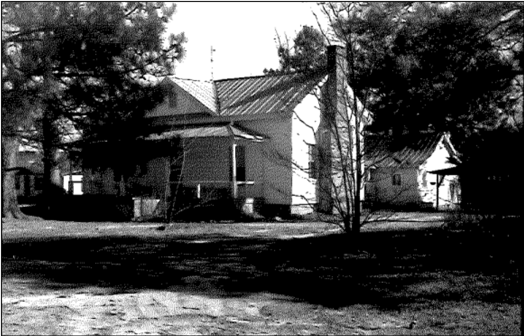
Figure 24. House, south side and west front elevations in 1990 (photographer: Kelly Lally)
