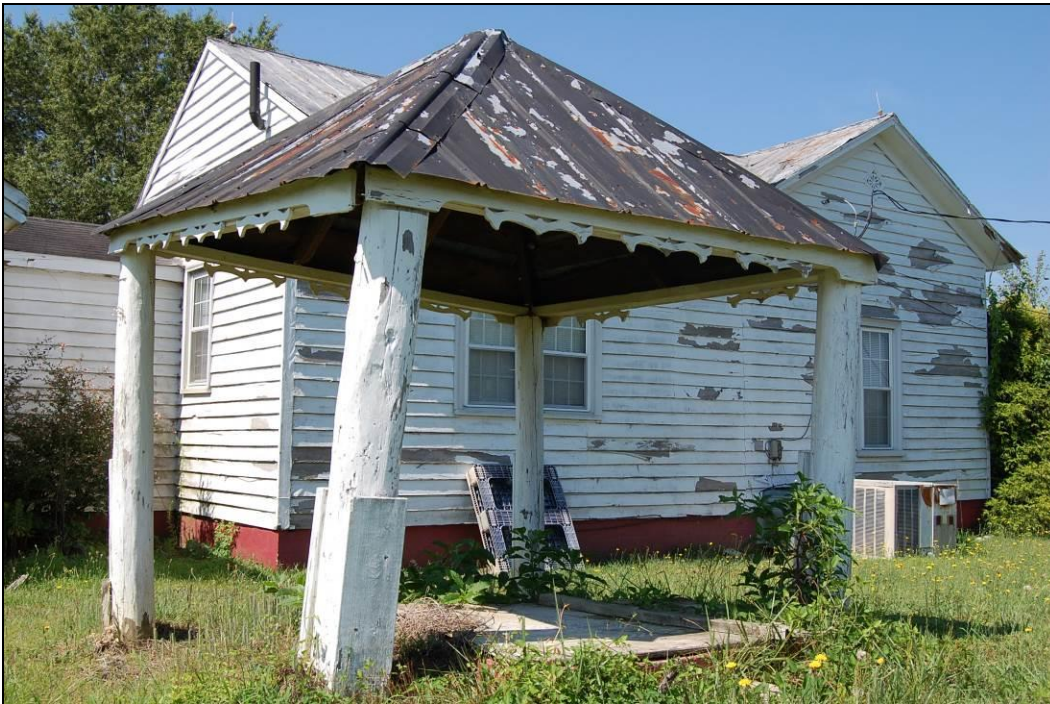
Figure 42. Looking southwest at well house and north side of house
