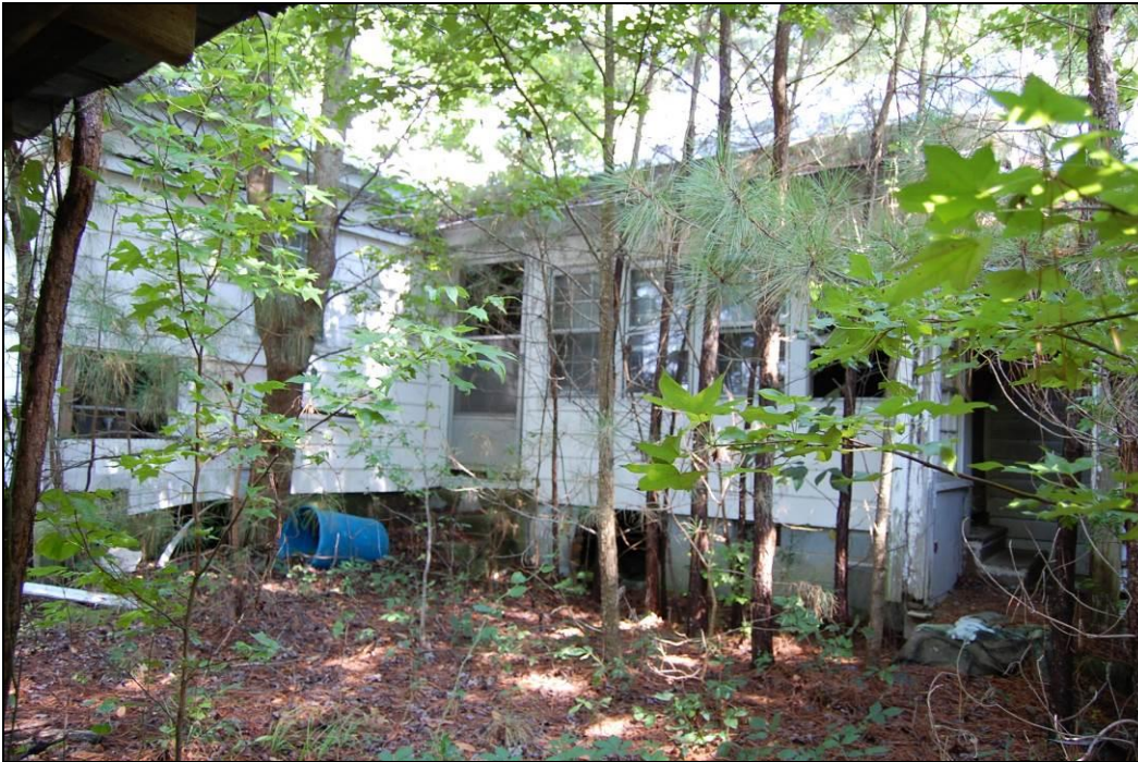
Figure 25. House, looking northwest at east rear elevation of main block at left and later-enclosed porch at south side elevation of original rear ell
