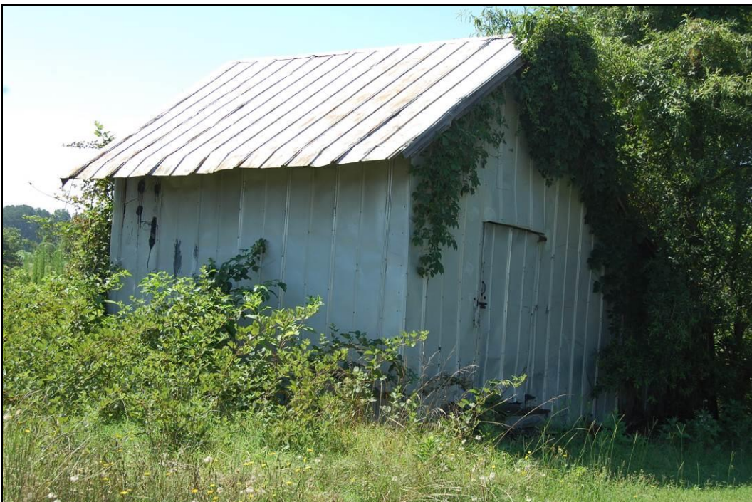
Figure 44. Looking southeast at shed
