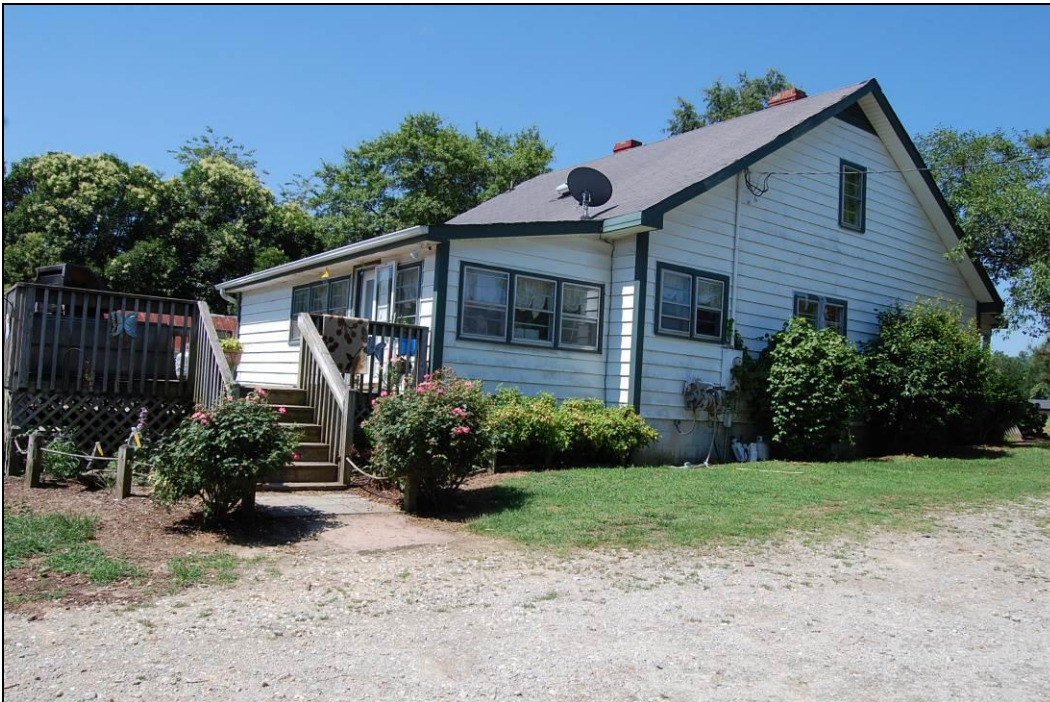
Figure 18. House, east rear and north side elevations
