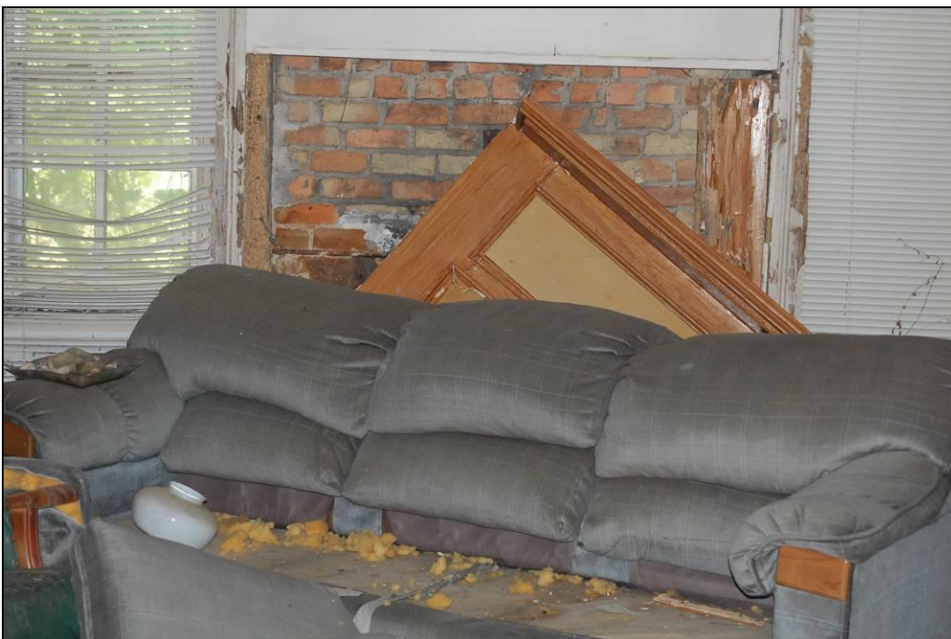
Figure 32. House, looking into north room from hall at detached mantel
