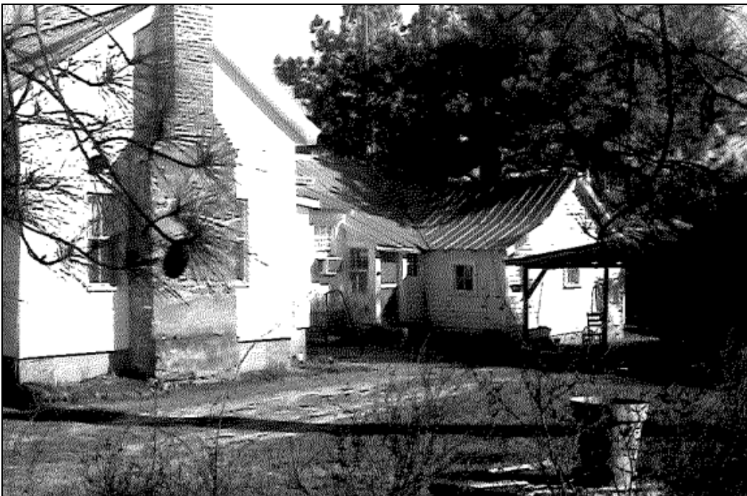
Figure 26. House, looking northeast at south side elevations of main block at left, original rear ell at center, and later east ell at right in 1990 (photographer: Kelly Lally)
