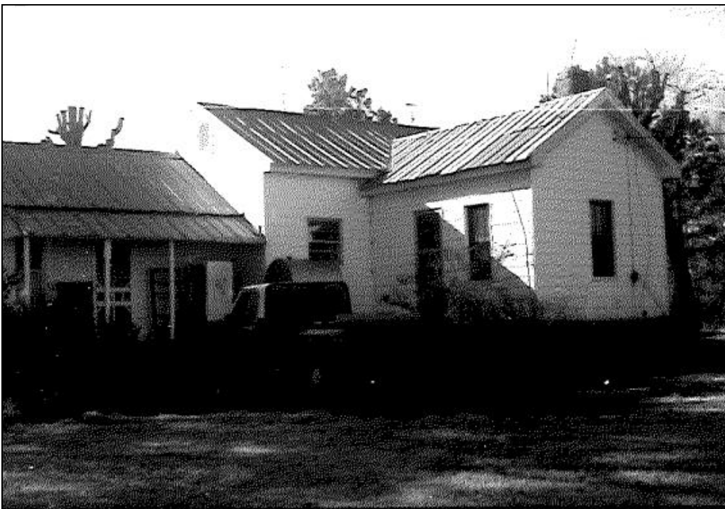
Figure 30. House, north side elevation of kitchen wing at left and original rear ell at center with later north addition at right in 1990 (photographer: Kelly Lally)
